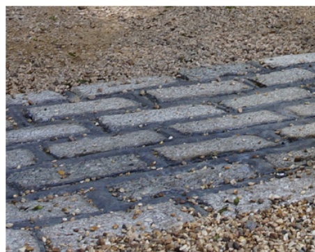
Stone sett thresholds
